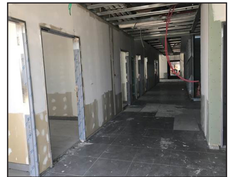
Interior hallway of the Well-Being Center facilities
